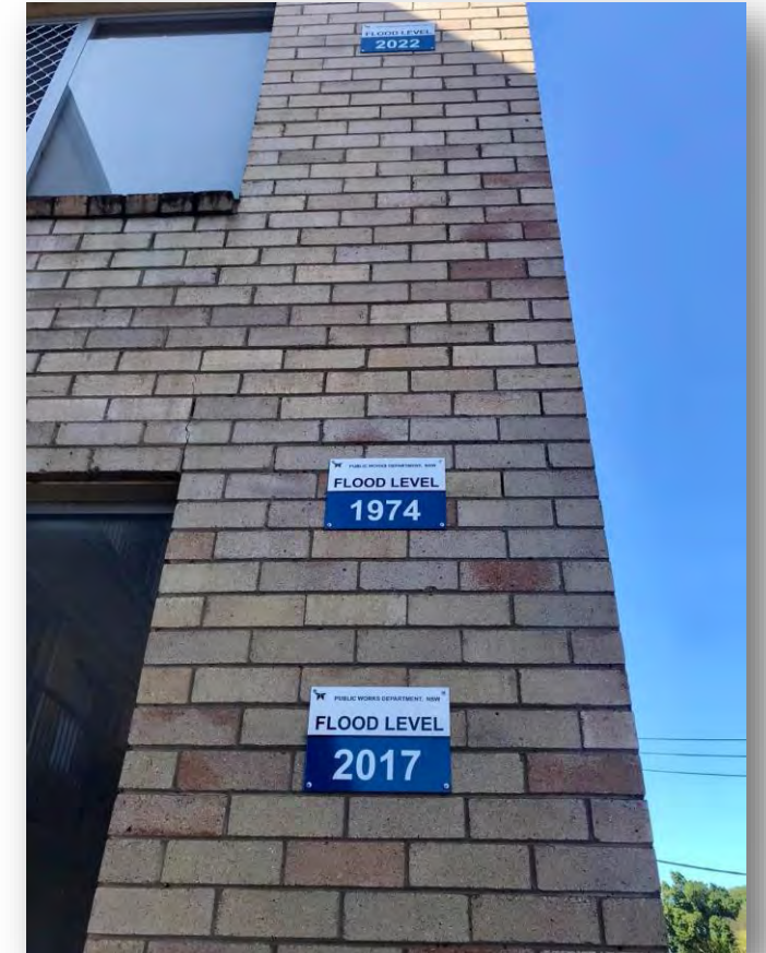
Flood level markers on Aza Motel, Lismore. Photo: Andy Gough
